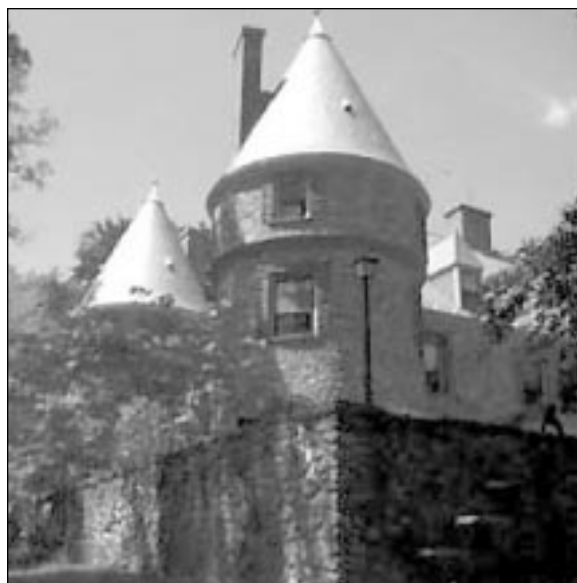
Above, the Grey Towers National Historic Landmark
